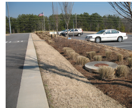
Figure 3.3-27 Parking lot bioretention in Johns Creek, GA.
