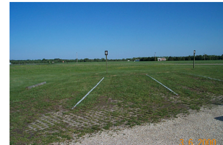
Figure 3.3-26 Permeable overflow parking area
