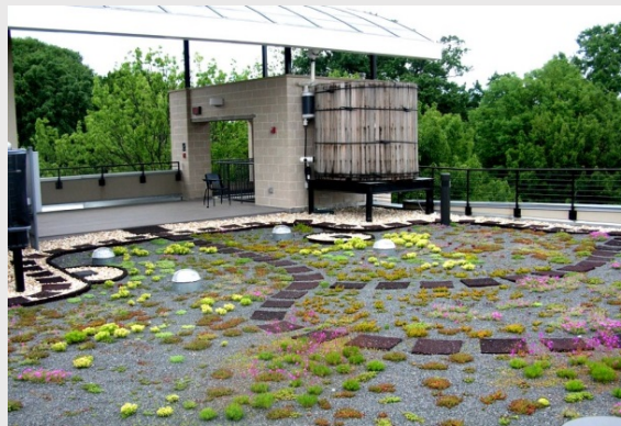
Figure 3.1-2 South Face Eco Office Green Roof (Source: www.vertical-theory.com )
