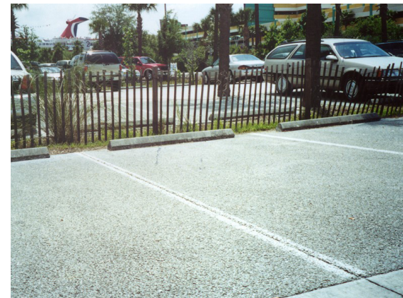
Figure 4.16-1 Typical Pervious Concrete System Applications (Photos by Bruce Ferguson, Don Wade)
