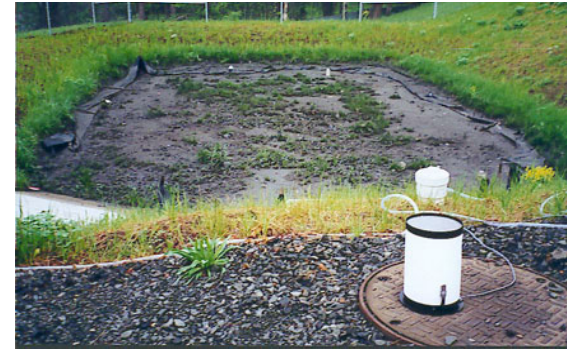
Surface Sand Filter
