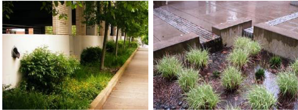
Figure 4.24-1: Various Stormwater Planters
