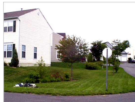
Figure 4.4-3 Bioretention Area in a Subdivision (Source: US EPA)
