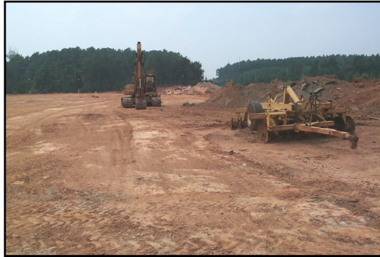
Figure 2.1.1-1 Clearing and Grading Alter the Hydrology of the Land
