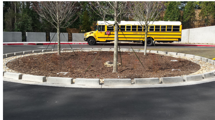
Figure 3.3-24 Cul-de-sac bioretention at E. Rivers Elementary School in Atlanta.
