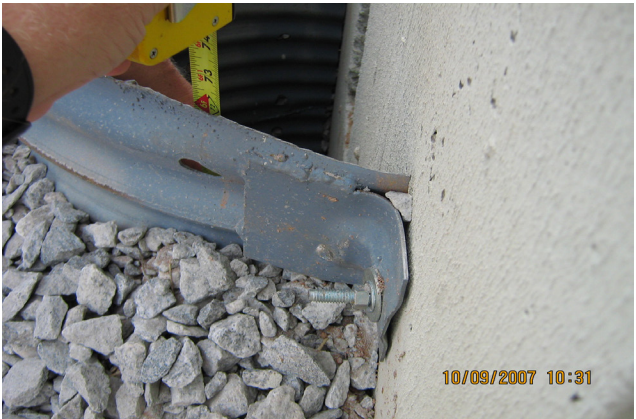
Figure 2. Affixed to Concrete Structure
