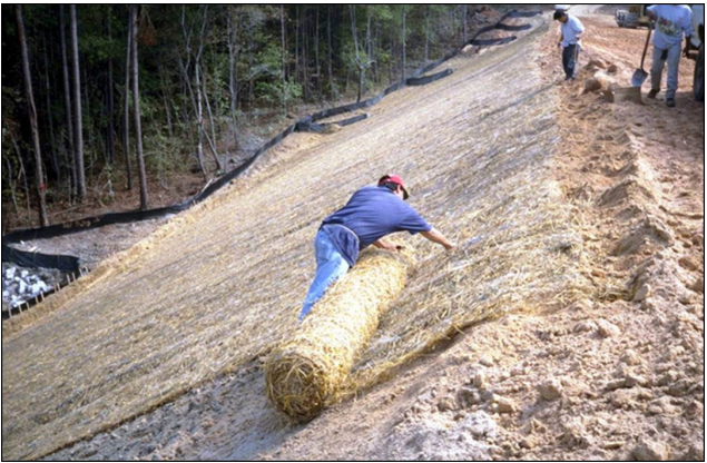
Figure 2. Installation of Jute Matting
