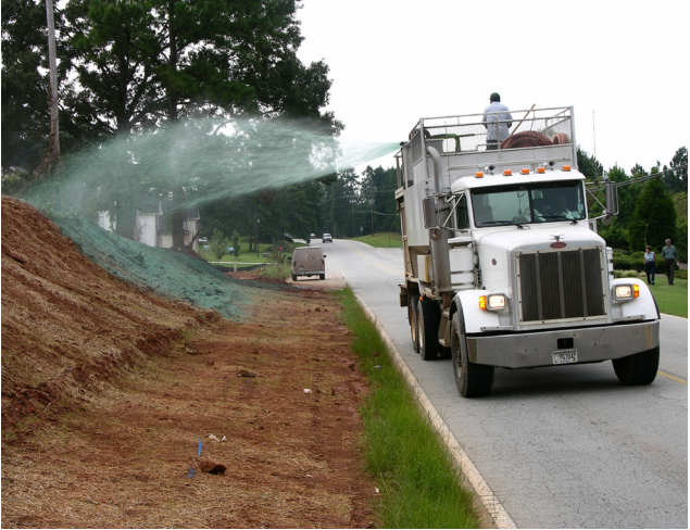
Figure 1. Hydroseeding on disturbed areas
