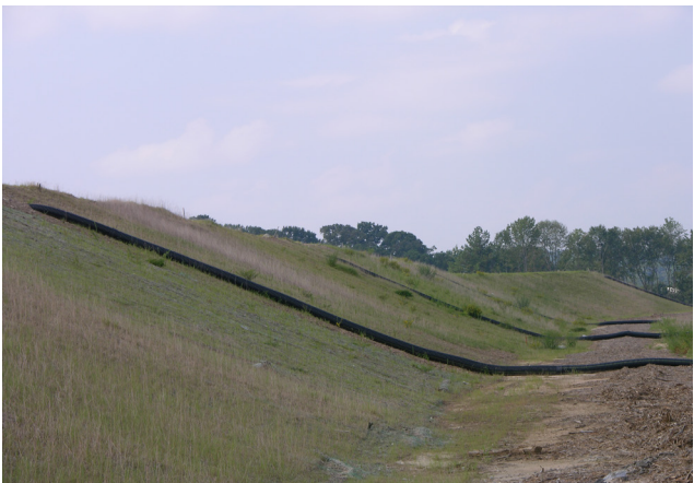
Figure 2. Diagonally Placed Downdrain
